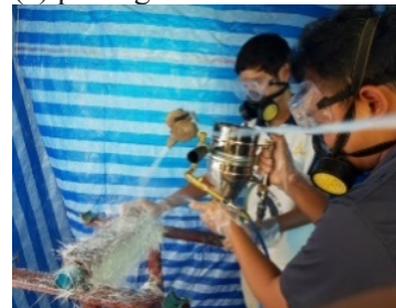
(b) spraying GFRP and resin
